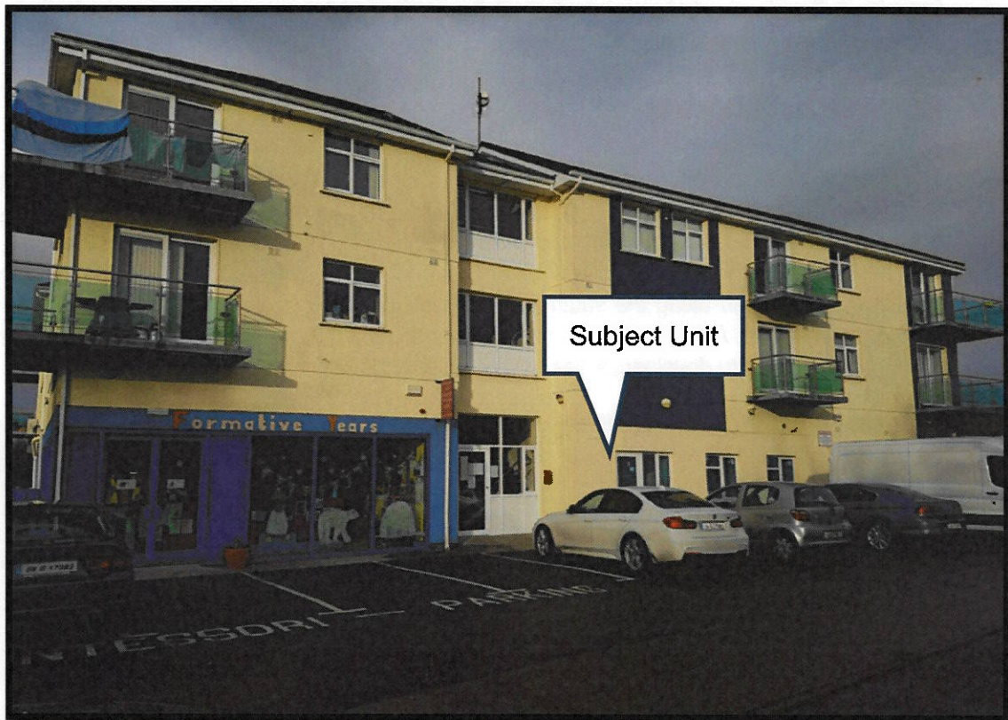
Figure 2: Photo (December 2018) showing the completion of the proposed external alterations to the building, which is materially different to the “shopfront” of the adjoining Creche.
